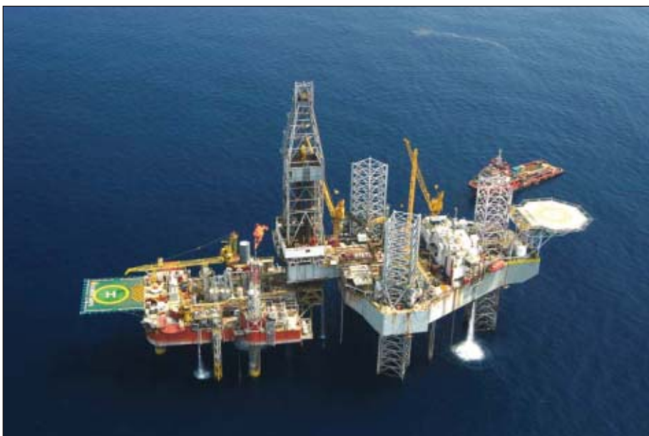
The Atwood Vicksburg jack up drilled the seven producing wells on the mat-supported mobile oil production unit in Cendor field off Malaysia (Fig. 2). Photo from Petrofac Ltd.
